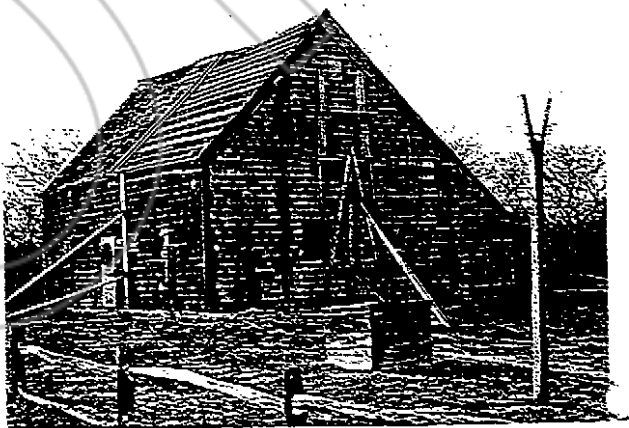
Figure 3. Buildings seriously damaged by storms or deterioration may need to be braced before architectural evaluations can be made. Jehro Coffin House. Photo: John Milner Architects.
