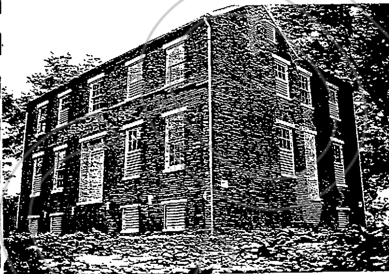
Figure 1. Proper mothballing treatment: This building has been successfully mothballed for 10 years because the roof and walls were repaired and structurally stabilized, ventilation towers were added, and the property is maintained. Photo: Charles E. Fisher, NPS.
